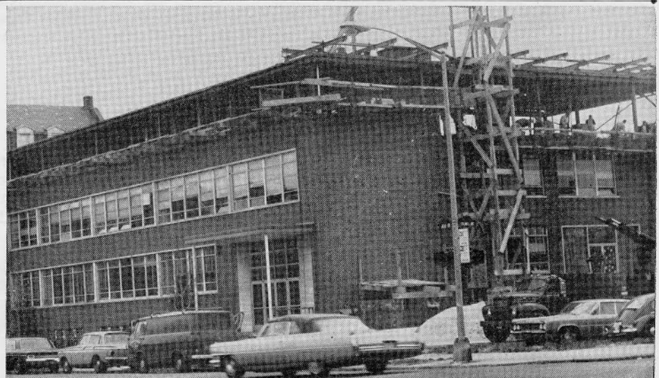
At right: A recent foto of the Yeshiva shows the third floor at the half-way mark. The steel beams and roof are up and the scaffolding for the brick layers is being prepared. Story on Page 2. Photo by Pixie
