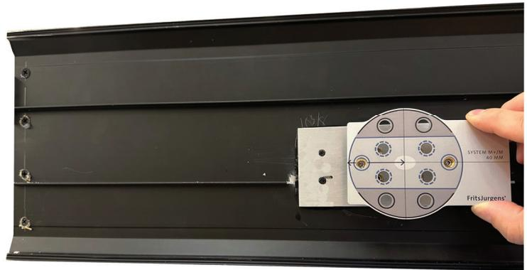
Use the metal template provided and measure the distance of the pins from the edge of the sill to find the placement of the holes in the floor.
