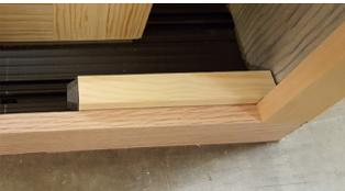
4 1/8" Bumper applied to bottom and top of interior sill and head jamb opposite of primary panel with handle set.
