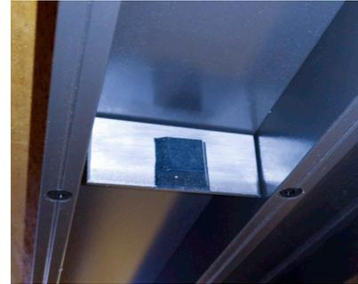
Use screws to apply pocket stops **FIG 13**. These must be removable in the event that future service is required on this unit.
