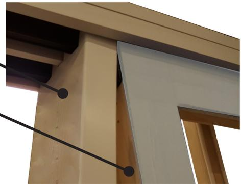
**BEFORE INSTALLING ACTIVE PANELS, REMOVE THE INTERIOR HEAD JAMB STOP AND PARTING BEADS IN THE HEAD JAMB.**
